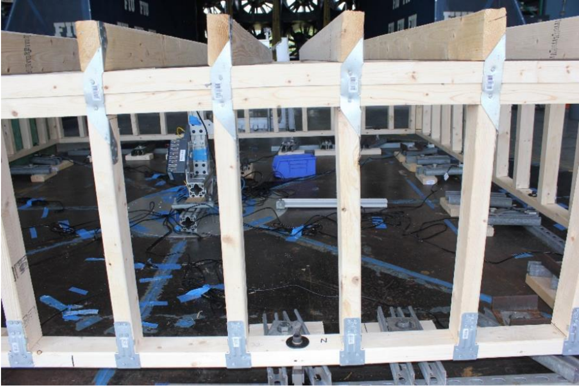
Figure 14: Connectors at roof-to-wall and wall-to-foundation interface
