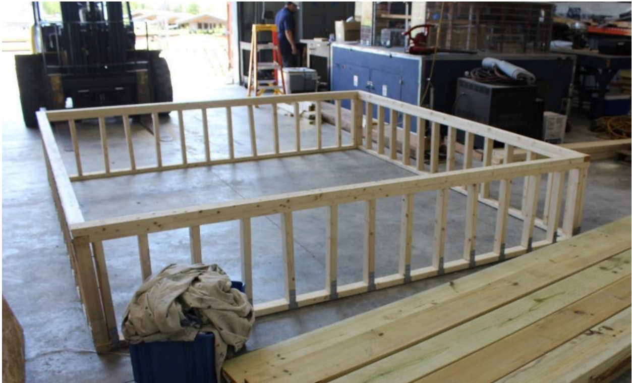
Figure 3: SSM model walls constructed
