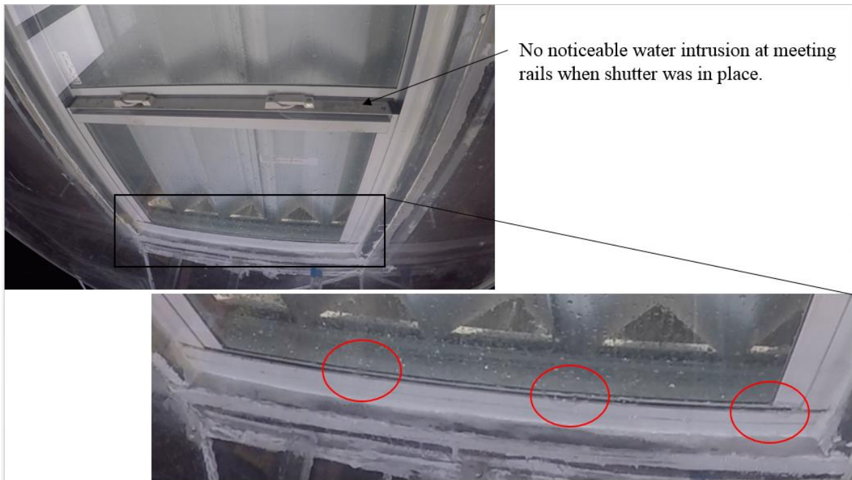
Figure 13 Observed water intrusion through the nonimpact window with the accordion shutter installed (62 mph).
