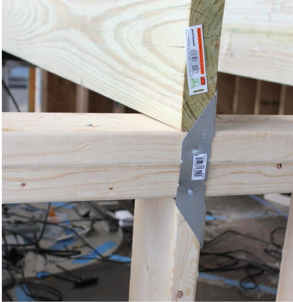
Figure 16: ST-H2A connector at joist-to-top plate / top plate-to-stud, typical
