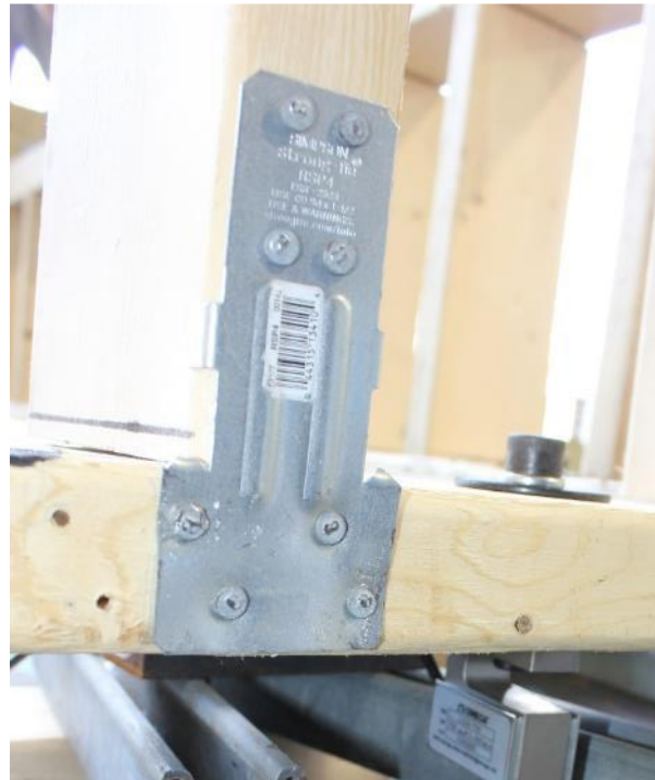
Figure 15: ST-RSP4 connector at stud-to-bottom plate, typical
