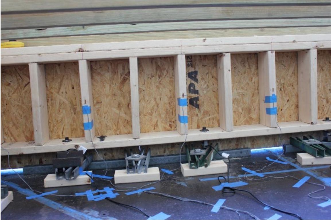
Figure 19: Load cells and strain gages installed on FSM model
