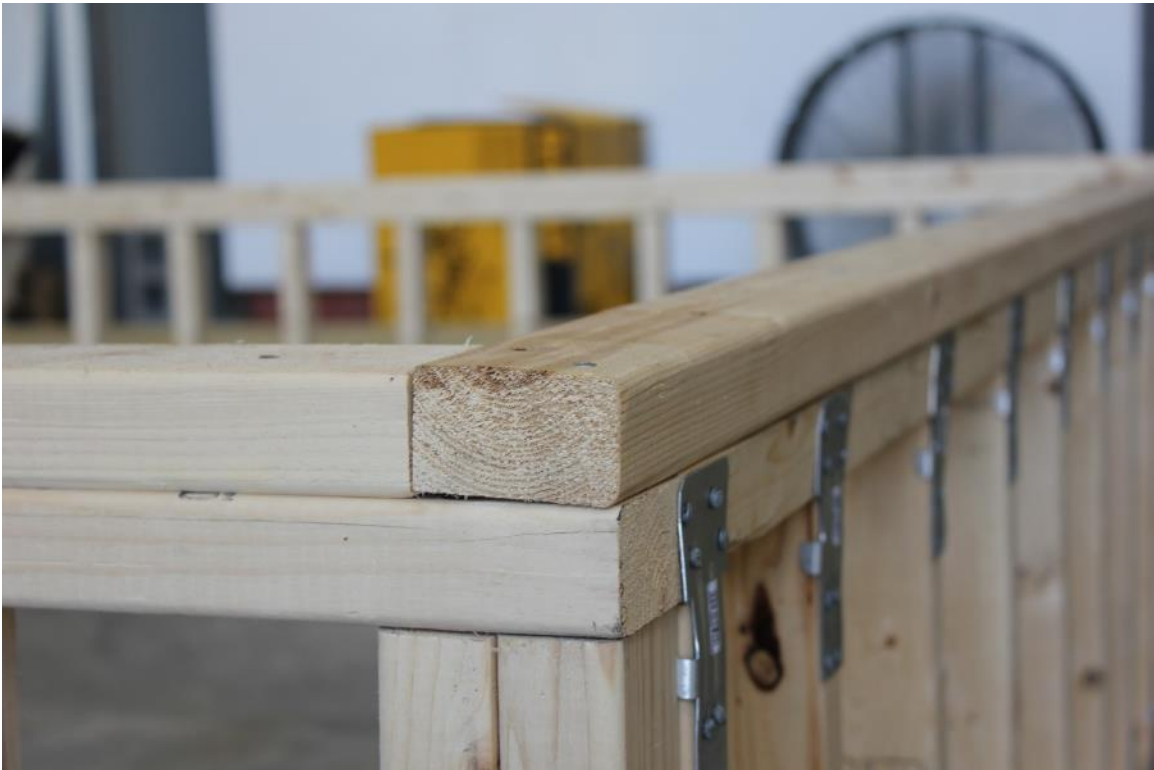
Figure 5: Top plate lapping at corners, typical
