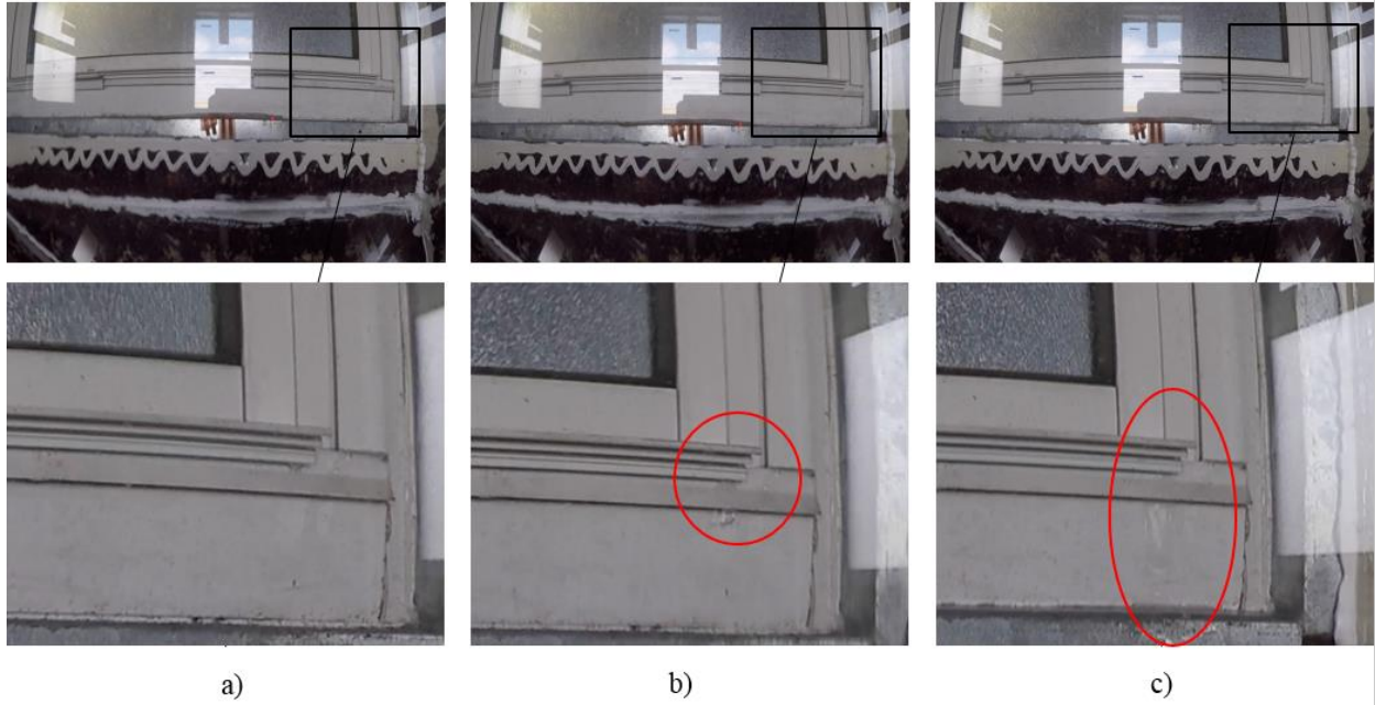
Figure 12 Observed water intrusion through the impact-rated window (62 mph, 0° wind direction): a) prior to water intrusion, b) water intrusion commencement, and c) steady flow of water intrusion for remainder of test.
