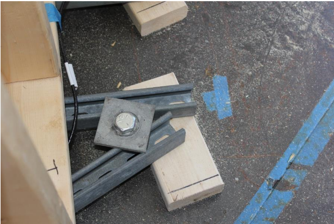
Figure 18: Uni-struts anchored to ground w/ anchor bolt
