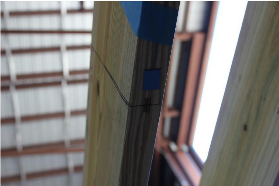
Figure 20: Strain gage attached to roof joist
