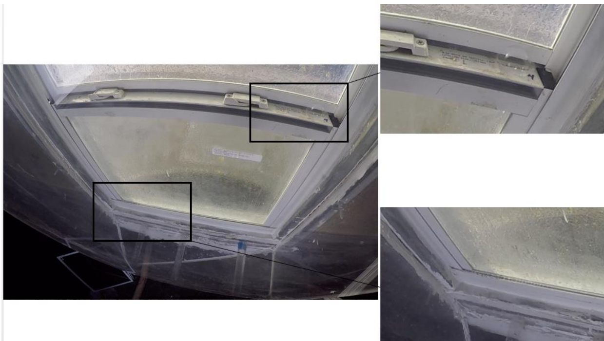
Figure 11 Observed water intrusion through the nonimpact window (62 mph, 0° wind direction).
